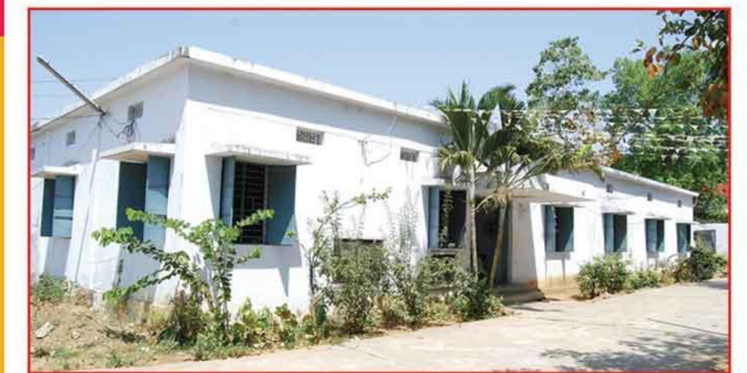
Manochaithanya Vocational Training Centre Building
